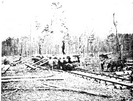
FIG. 121. — Loading Log Cars with a Crosshaul. Missouri.
